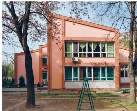
The load bearing structure is in the reinforced concrete frame system with exposed beams and pillars. The ribbed floor slabs have straw ceilings, while above the hall there are wooden trusses of the pitched roof. The facade walls with visible brickwork are uninsulated. The windows are wooden, single-framed connected double sashes, while the metal fenestration in the entrance halls and hallways is without thermal breaks. The floors are also without thermal insulation.
