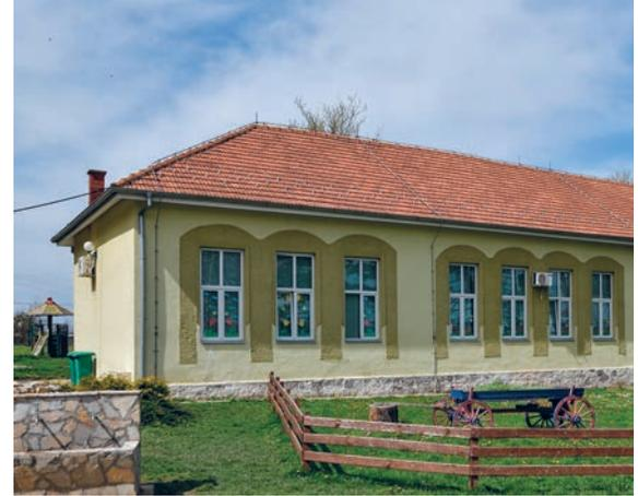
Kindergarden facilities of this type were built using simple traditional construction techniques. The load bearing structure is massive, with a basic wooden construction to the unheated attic, and a hip roof. The facade walls are plastered on both sides, with plain decorative plasterwork on the exterior and without thermal insulation. The windows are wooden framed, double-sashed with single glazing. There is wood flooring without thermal insulation.
